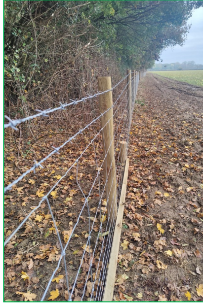
Stock fencing with 2 strands of Barbed Wire: fencing along Kinsham Lane, fencing along southern boundary of reserve, fencing along edge of South Ride up to public footpath
