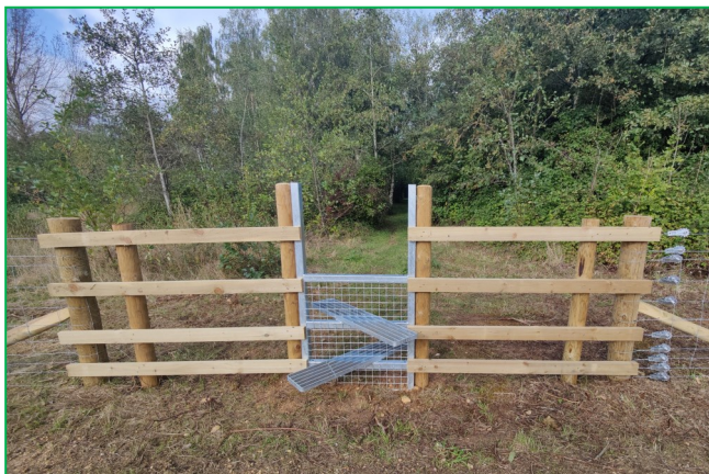
Metal Shetland Stile: stile in position on public footpath
