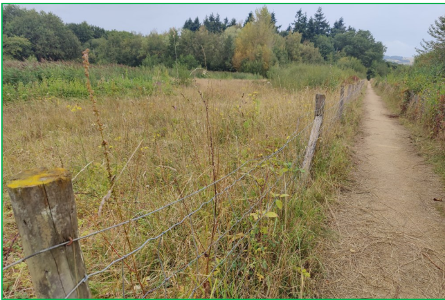
Stock fencing with 2 strands of plain wire: old fencing along public footpath before removal, new public footpath fencing
