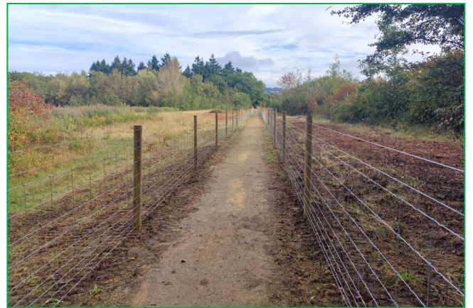
Stock fencing with 2 strands of plain wire: old fencing along public footpath before removal, new public footpath fencing
