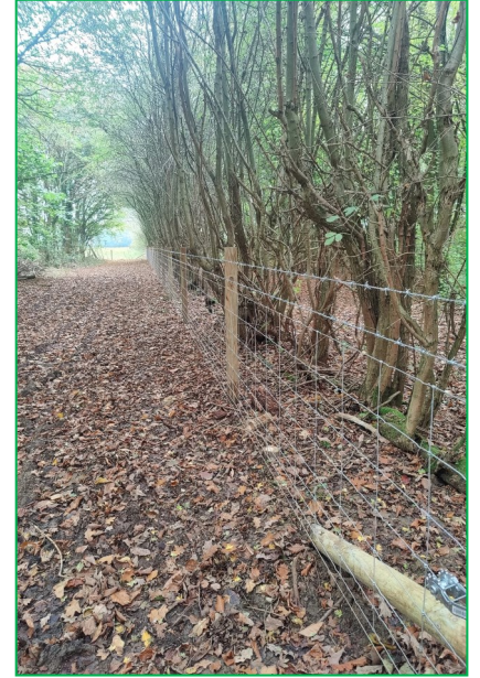
Stock fencing with 2 strands of Barbed Wire: fencing along Kinsham Lane, fencing along southern boundary of reserve, fencing along edge of South Ride up to public footpath
